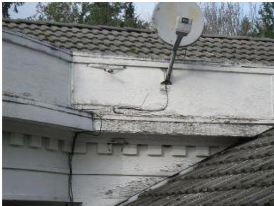
Exterior Surface: Siding deterioration on west side
