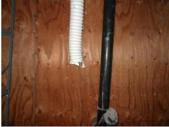
Crawl Space: Dryer venting to crawl space
