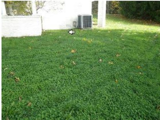
Grading / Drainage: Negative slope near A/C unit
