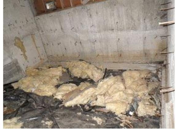
Crawl Space: Insulation falling down underneath south sun room
