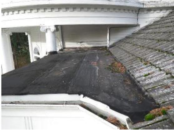
Roofing: Torch Down roofing
