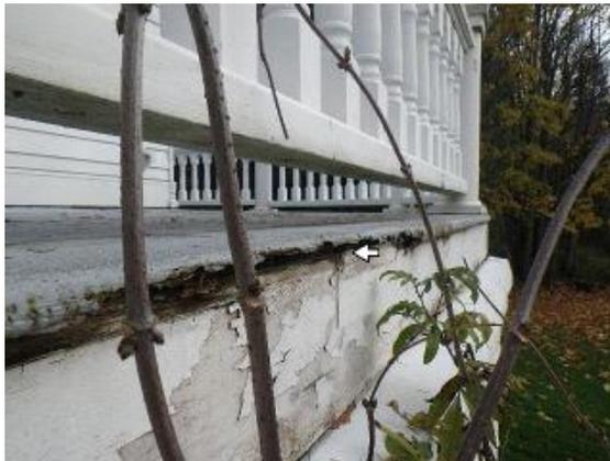
Decks / Balcony: Deterioration noted in bull nosing
