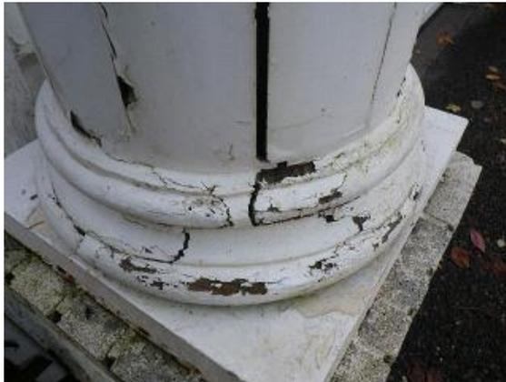
Garage/Carport: Column on garage corner showed signs of deterioration.
