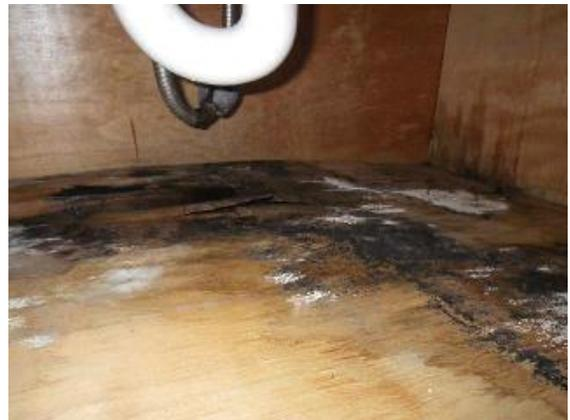
Laundry Facilities: Deterioration from past plumbing leaks
