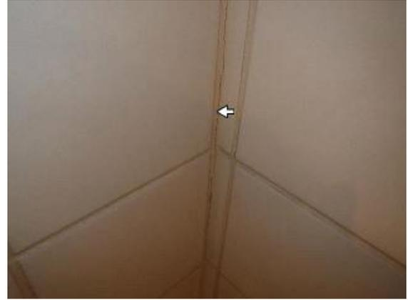
Bathroom 1: Caulk deterioration in shower
