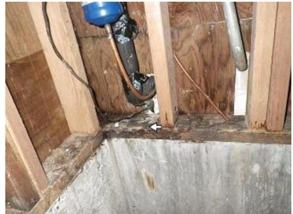
Under Floor Framing & Support: Wood deterioration in framing and sheeting at A/C penetration- southwest corner.
