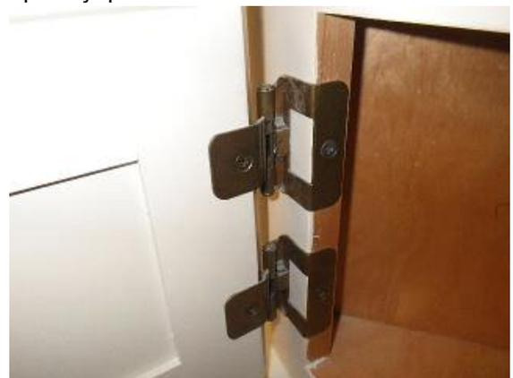
Bathroom (master): Cabinet door on side of tub loose
